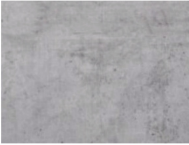
5. EXTERNAL CONCRETE WALLS
